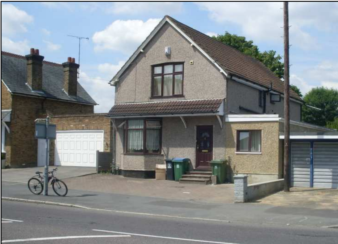
House after conversion and extension
